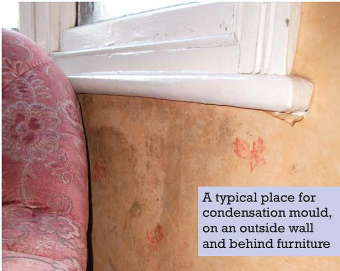
A typical place for condensation mould, on an outside wall and behind furniture
