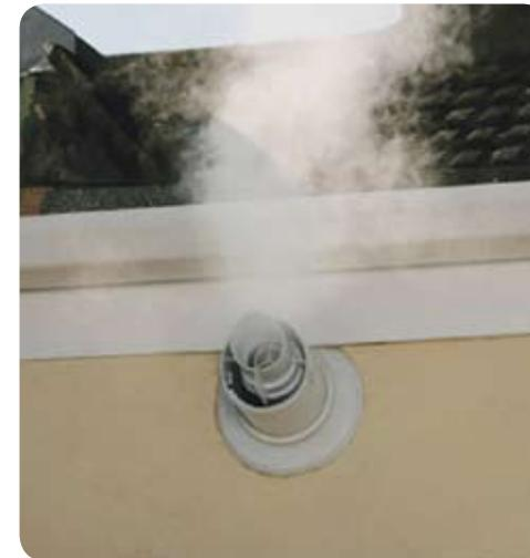
While old non-condensing boilers convert around 60% of their fuel into heat (SEDBUK G-rated boilers), the efficiency rate of modern SEDBUK A-rated condensing boilers is at least 90%.
